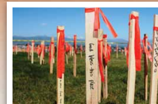
May 22, 2005, groundbreaking day for the Atrium and The Chapel. People wrote personal prayers on wooden stakes driven into the ground as a blessing on the construction site.
